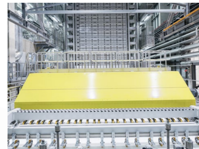
The mill is a complete ANDRITZ turnkey operation.
