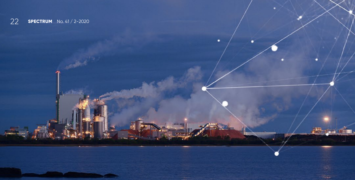
The first Metris DryQ solution is installed at the Montes del Plata mill in Uruguay.
