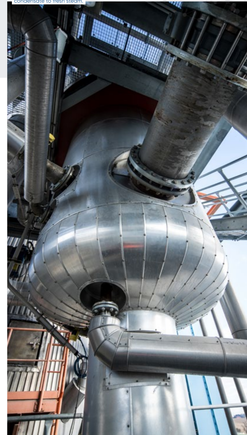
Vapor reboiler converts clean condensate to fresh steam.
