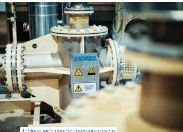
T-Piece with counter pressure device
